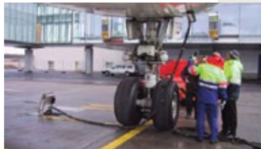
400Hz electrical power supplied through in-ground services pits at gates or remote stands.
